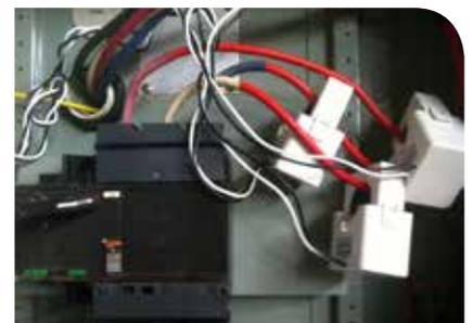
Figure 1 CT clamps on dairy shed circuit
