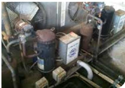
Figure 5 Vat compressors. Monitoring identified that one was running but no cooling effect
